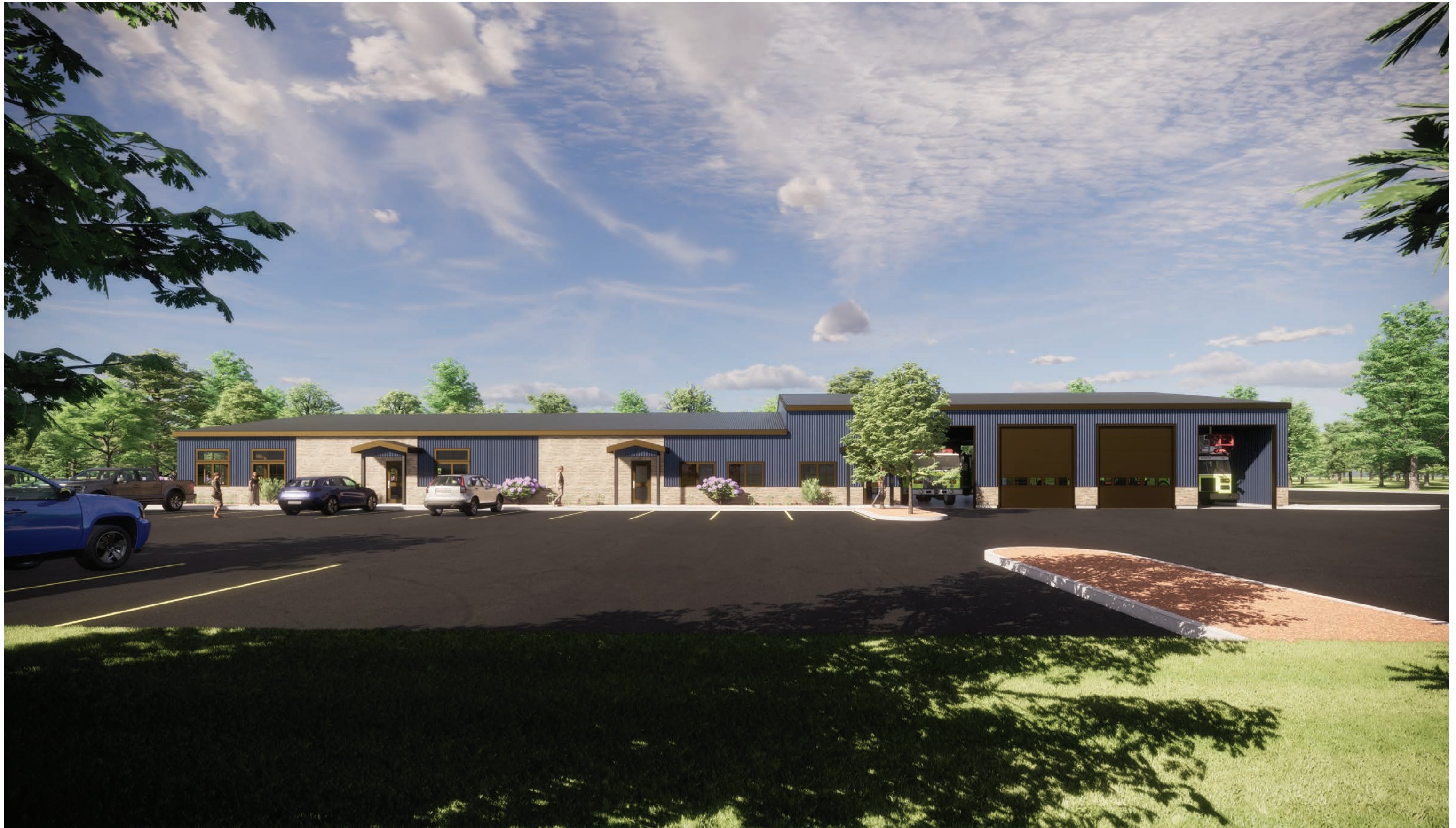
BEAR CREEK TOWNSHIP FIRE HALL
